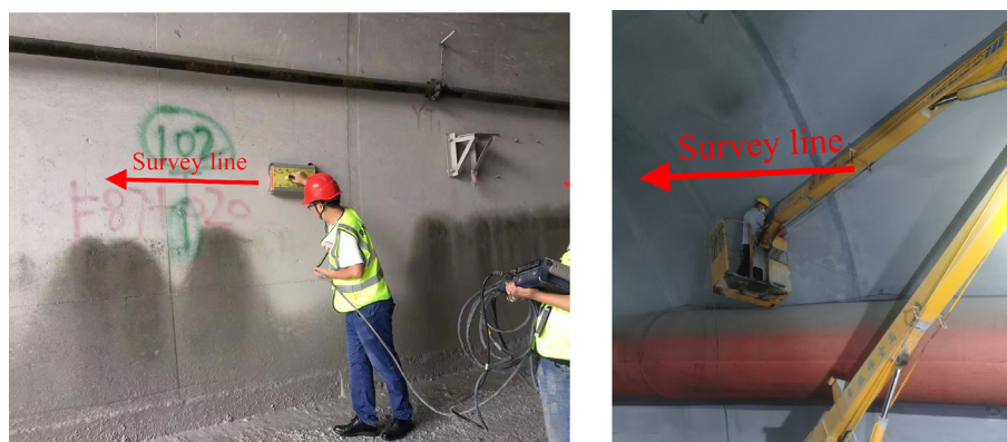
Fig. 6. GPR data acquisition in a rock tunnel.
