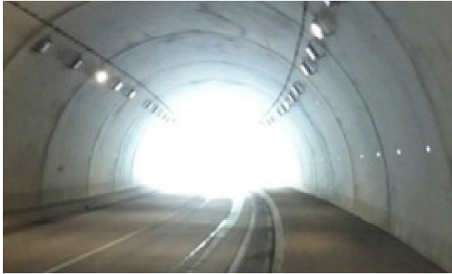
Fig. 3. White-hole effect near the tunnel exit.
