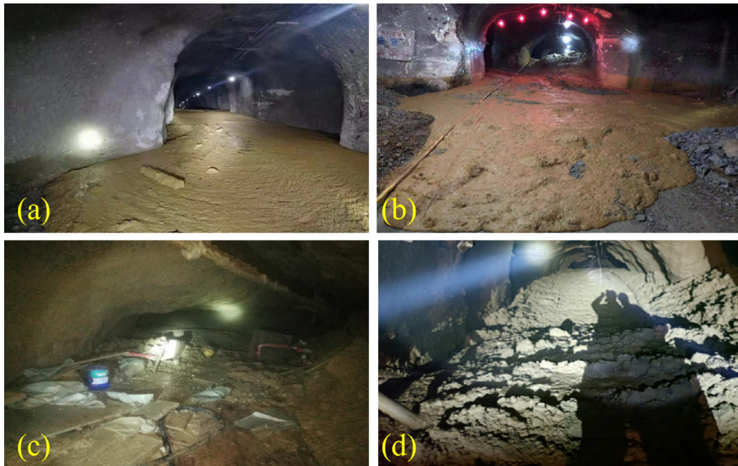
Fig. 4. Underground debris flow burying the tunnel. (a) August 2019, (b) November 2019, (c) underground debris flow destroying mining facilities, and (d) underground debris flow leading to ore dilution.
