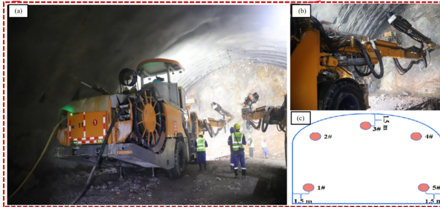
Fig. 9. (a) T31Y integrated multi-function rock drilling rig, (b) horizontal drilling operation process, and (c) drilling layout diagram.
