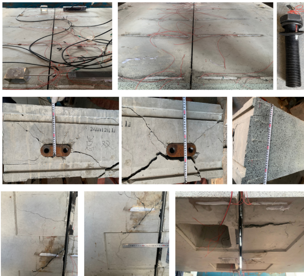
Fig. 22. Cracking pattern of DRSJ.
