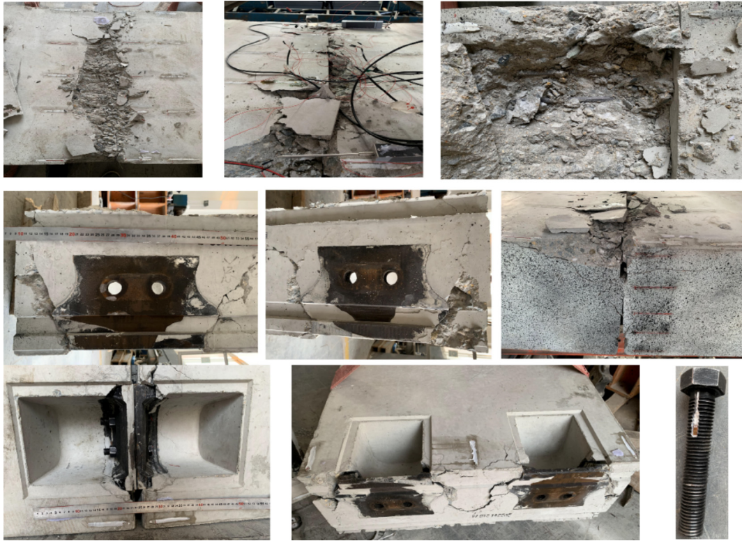
Fig. 20. Cracking pattern of CIJ.
