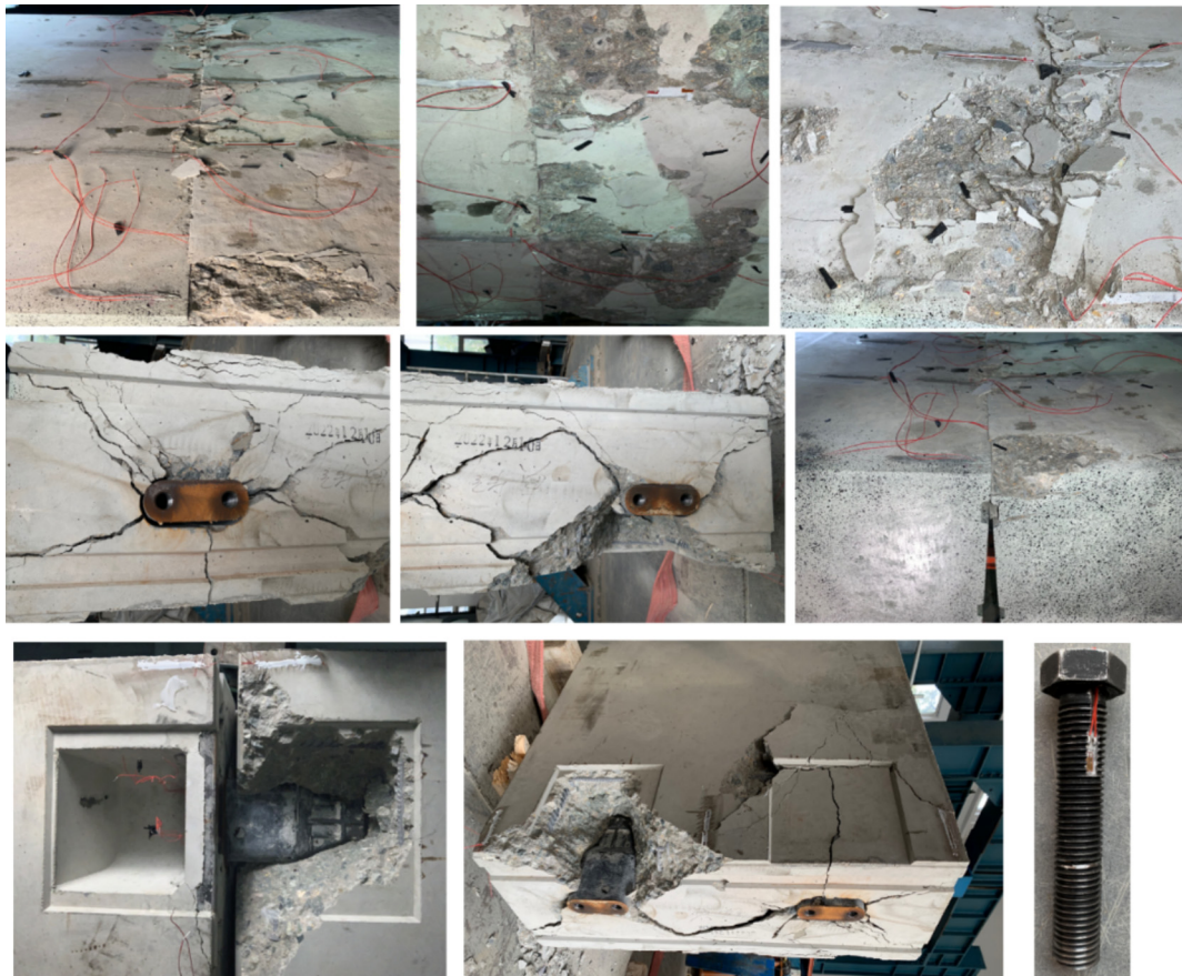
Fig. 21. Cracking pattern of SRSJ.
