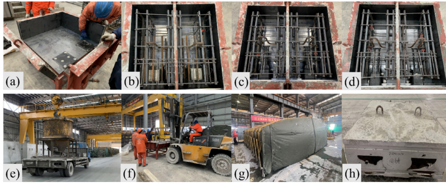
Fig. 2. Construction stages of shield tunnel joints: (a) mold setup and surface preparation, (b) placement of CIJ and rebar, (c) placement of SRSJ with rebar, (d) assembly of DRSJ and rebar, (e) concrete pouring operation, (f) steam curing after initial set, (g) formwork removal process, and (h) final curing of concrete outdoors.
