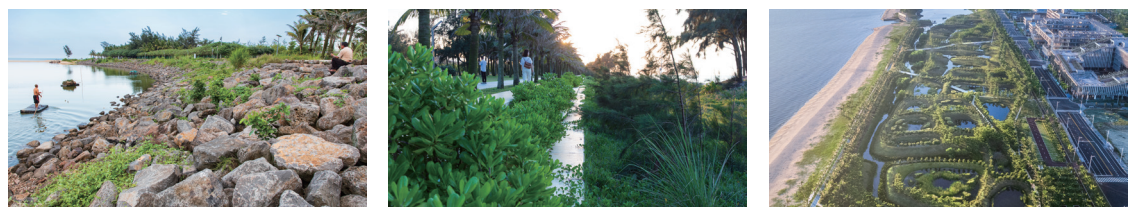
Transformed: breathing sea wall, spongy lush inland, and restored mangrove and native habitats
