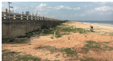
Pre-existing: a concrete sea wall exacerbated soil salinization, damaging the vegetated and amplified erosive forces
