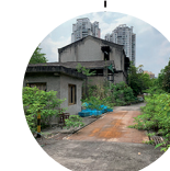
小锅炉房 Small boiler house
