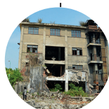
大锅炉房 Large boiler house
