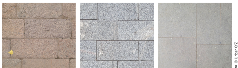
8. Photos of different paving patterns of granite: naturally-cleft, flamed, and bush-hammered, from left to right.
