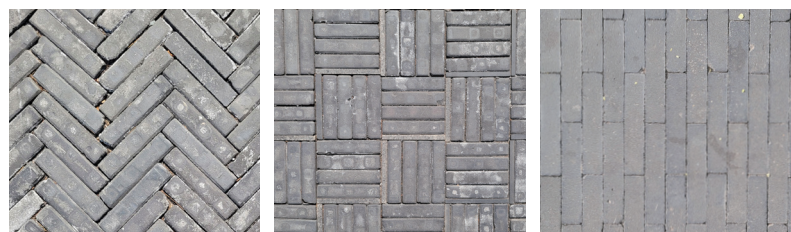
9. Photos of different paving patterns of brick: herringbone 45°, basket-weave, and stretcher-bond, from left to right.
