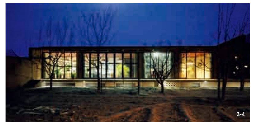
3. 工作室西立面春、夏及冬日景象。 3. The sceneries respectively in spring, summer and winter of the west facade.
