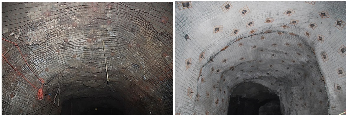
Fig. 10. Examples of Type 1 GDS system that were used in two Canadian metal mines.
