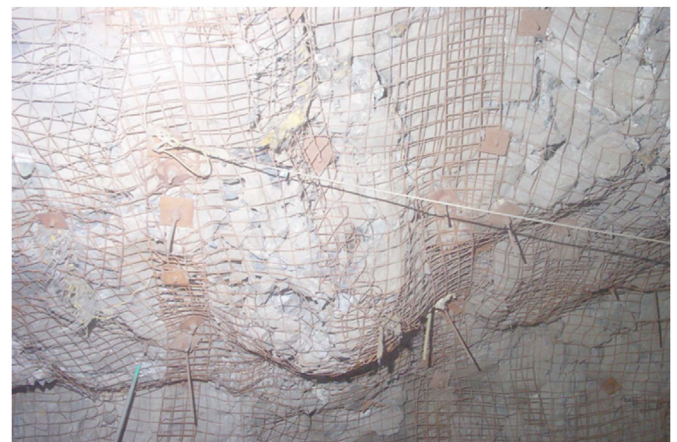
Fig. 3. Example of a strain-type rockburst mechanism, showing surface damage contained by the installed bolts and mesh ground support system in the roof of a mine excavation.
