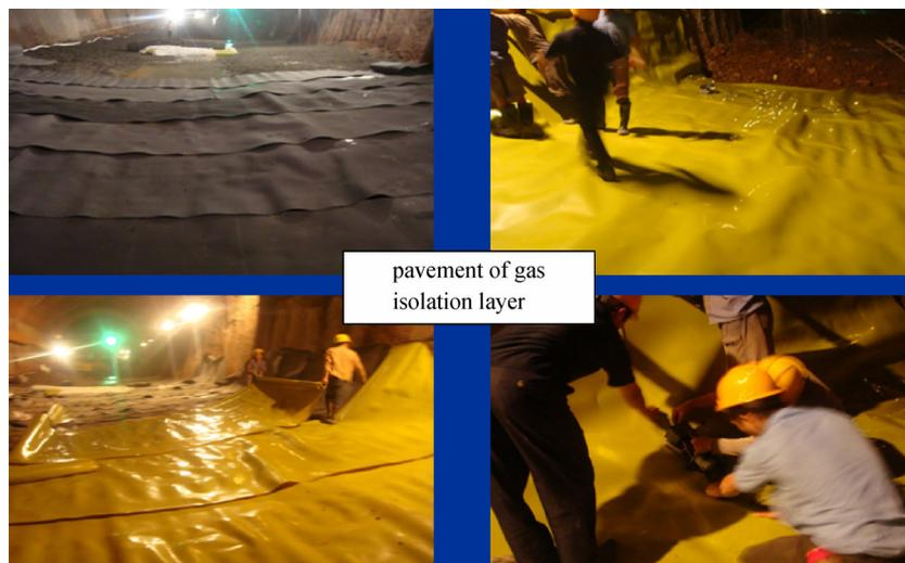
Fig. 6 Construction of gas isolation layer
