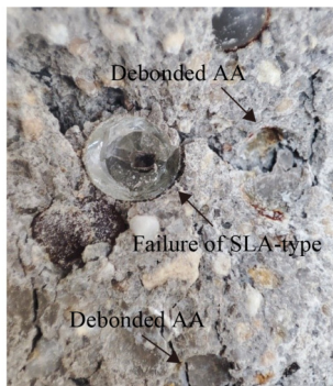
Fig. 9 The appearance of concrete failure surface after the compression test.
