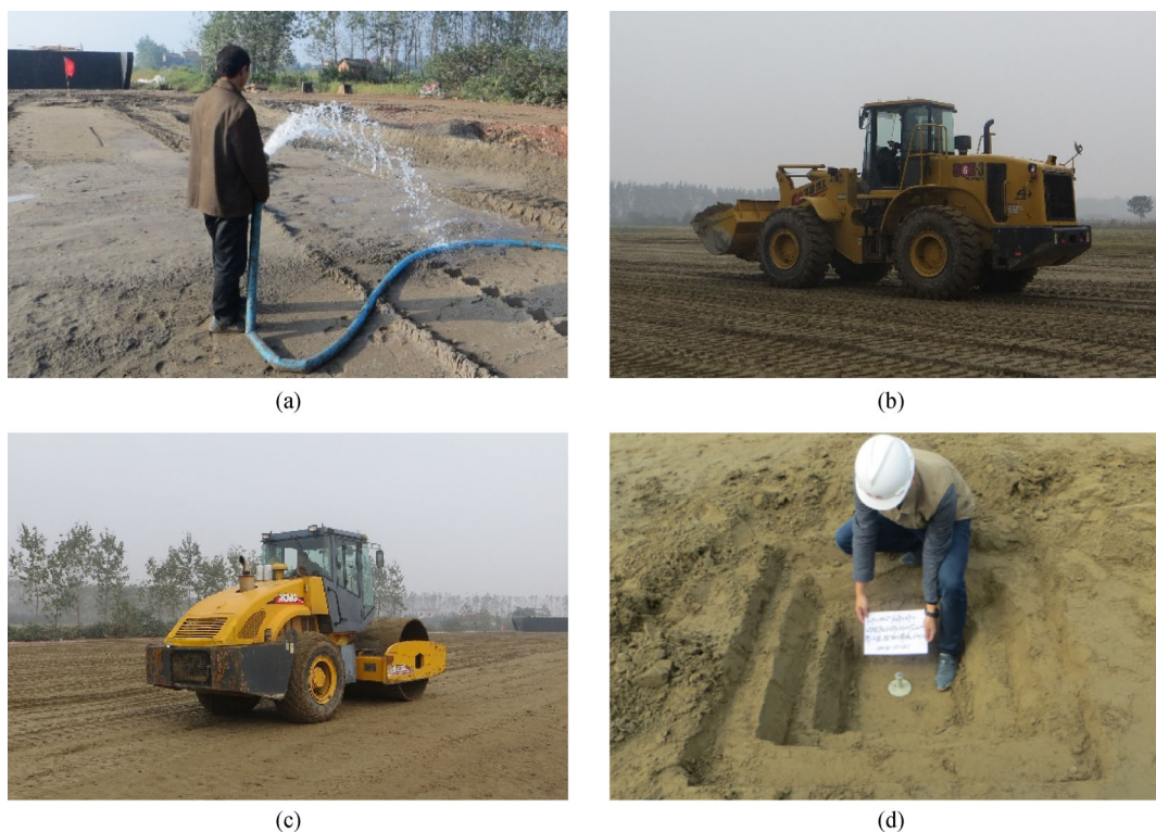
Fig. 2 Construction process of embankment using large thickness sand filling technique
