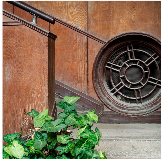
Fig. 20 The ventilation opening of the projection room.
