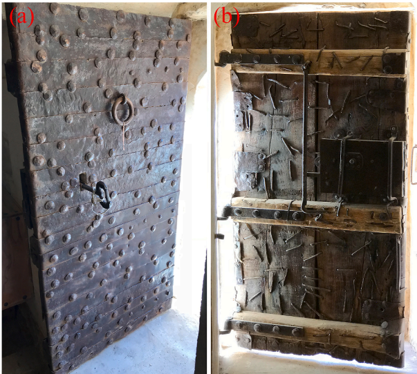
Fig. 10 Door leaf with metal riveted front face (a), Latch lock/kapazlama lock (b).
