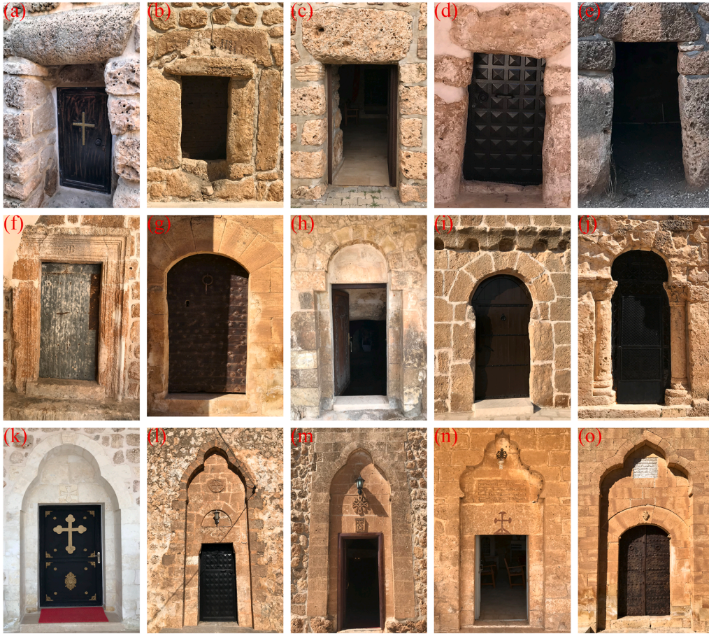
Fig. 9 Church entrance doors.
