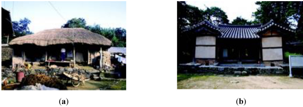
Fig. 1 Roofs made of straw and tiles for traditional Korean residences: (a) A typical three-bay straw roof house; (b) A tile roof house with ondol rooms and maru (Jeon, 2016).
