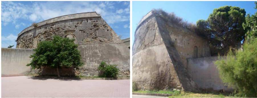
Fig. 4 The current state of the Tower (from Zerlenga et al., 2016b).
