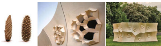
Fig. 18 Architectural applications of plant-inspired shape-changing interfaces: pine-inspired humidity-responsive architecture facades adjust light transmission for energy efficiency. Reprinted from Menges and Reichert (2015), Copyright 2015, with permission from John Wiley & Sons, Ltd.
