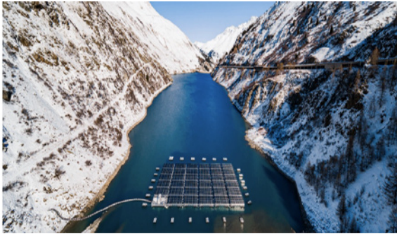
Fig. 14 448 kWp FPV at an altitude of 1800 m in Lac des Toules (adapted from Ref. [109] under the terms of CC BY license).
