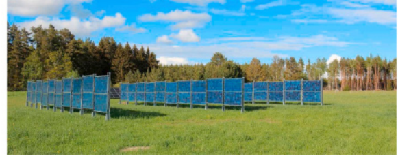
Fig. 8 Vertically mounted bifacial APV system in Sweden (adapted from Ref. [60] under the terms of CC BY license).
