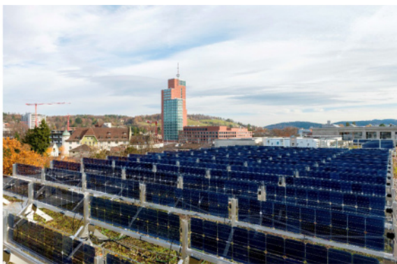
Fig. 9 Example of a vertically mounted BPV system on a green roof in Winterthur, Switzerland (adapted with permission from Ref. [79]).
