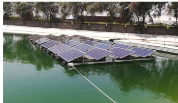
Fig. 13 Floating bifacial and monofacial system in Catania, Italy (adapted with permission from Ref. [108]).
