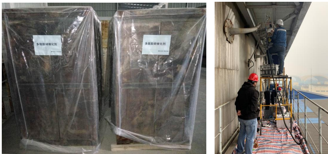
Fig. S1 Modified catalyst modules and sampling ports
