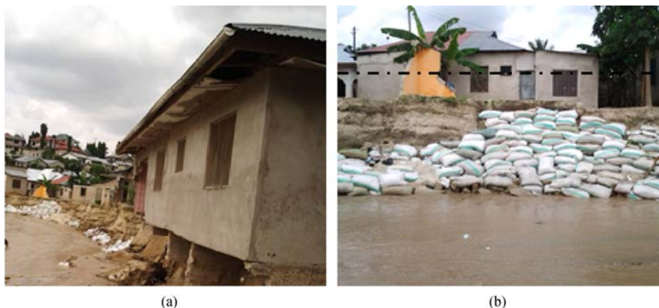
Fig. 9 Impacts of fluvial floods in the Kawe Ukwamani area. (a) shows some of the endangered buildings. (b) shows some of the community coping strategies against floods. The black line in (b) shows the height of the flood marks.
