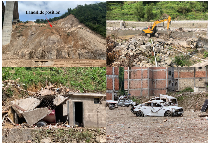
Fig. 2 Photographs of the disaster investigation field in Shanzao village, Yongjia county (Cong ZHOU, 2019-08-28 took photos). The red arrows indicate the position of the landslide.
