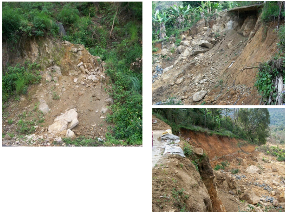
Fig. 2 Partial view of debris flow on a private plantation along the selected road stretch in 2014.
