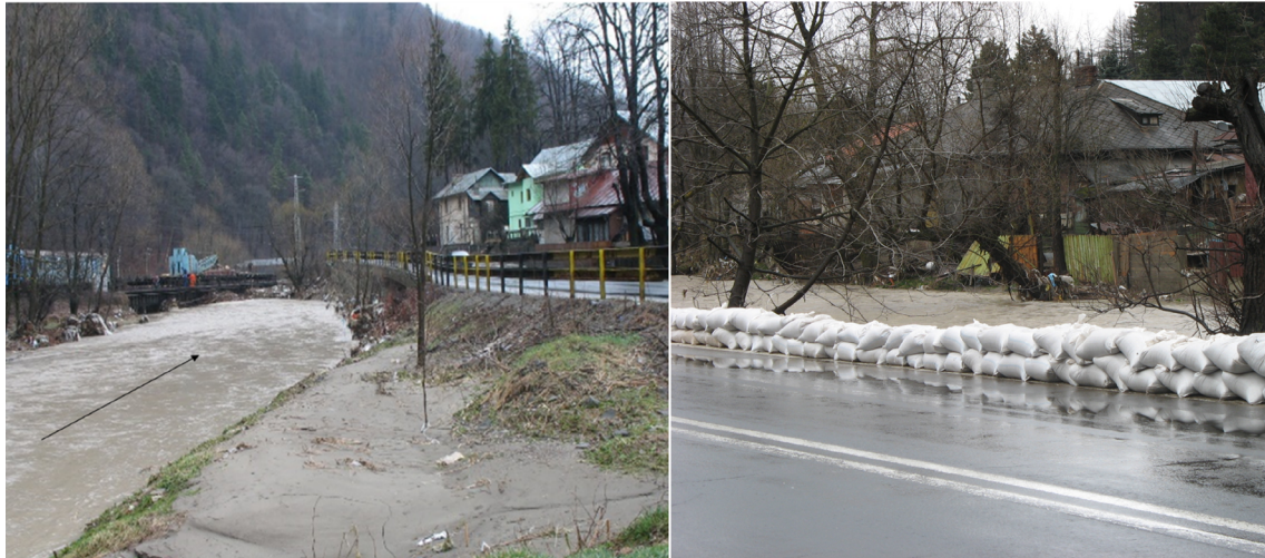
Fig. 8 Transport infrastructure (the national/European road DN1/E60 and railroad) and buildings exposed to flood and flooding risk in the upper Prahova Valley, in city of Sinaia (pictures taken by Gabriela Ioana-Toroimac during the flood of March 2007).
