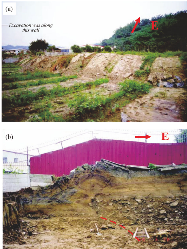
Fig. 6 Photographs of fault-related folding at the Wufeng excavation site. (a) The west-facing fault-related fold in the paddy field. (b) A cross-section of the Wufeng excavation site. The red dashed line is the main fault slip of the 1999 Chi-Chi earthquake ( M_w = 7.6 ) that occurred in Central Taiwan (Lee et al., 2001; Yang et al., 2014).
