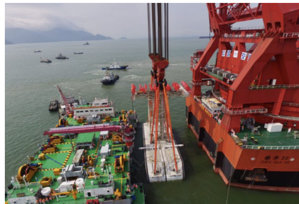
Fig. 4 Final joint installation of the immersed tunnel
