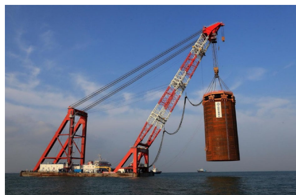
Fig. 2 Rapid formation of deeply inserted steel cylinder for the artificial island
