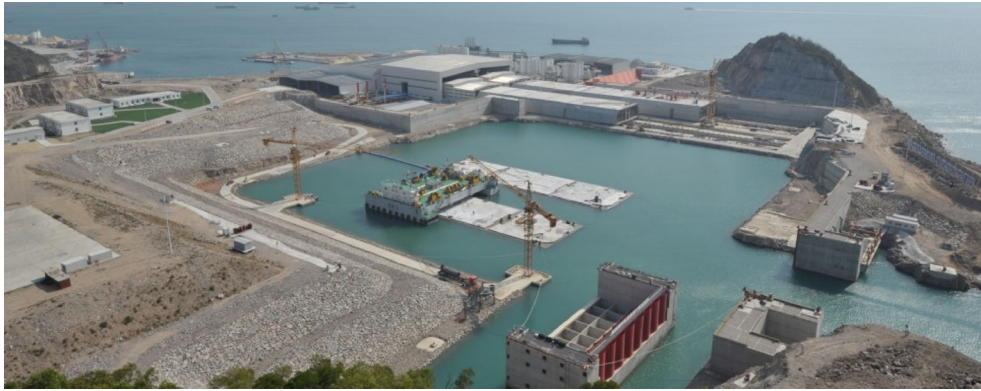
Fig. 3 Panorama of immersed tube precast plant
