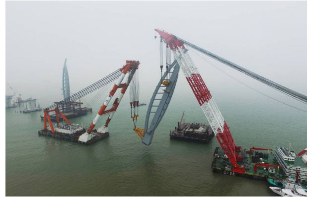
Fig. 6 Assembly construction of bridge structure
