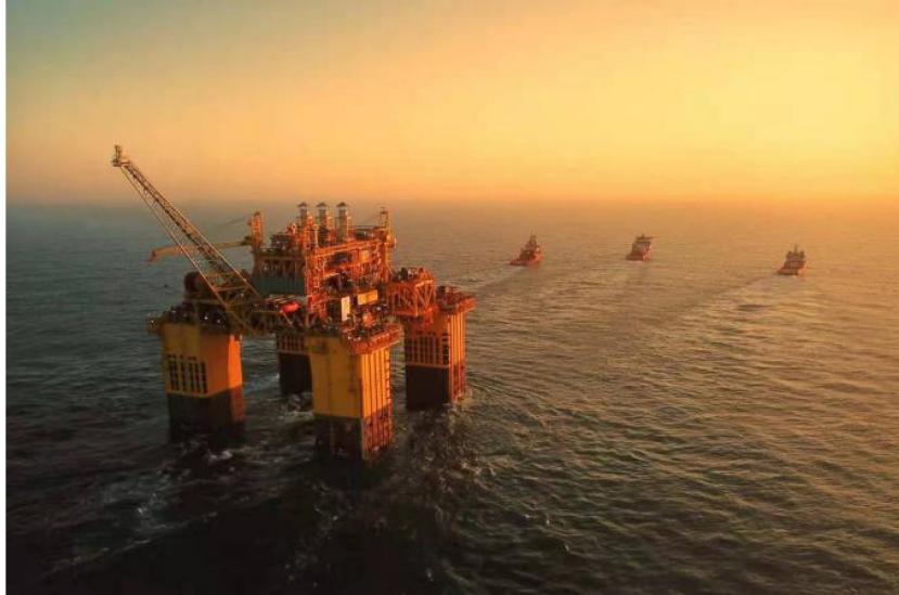
Fig. 5 Three-vessel wet-tow operation of the semisubmersible production and storage platform.
