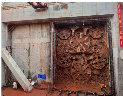
(a) Receiving of the left line rectangular pipe jacking machine
