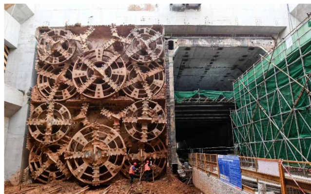
(b) Receiving of the right line rectangular pipe jacking machine
