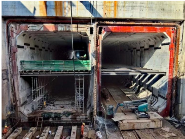
Fig. 12 Breakthrough of the twin tunnels at Shasan station.
