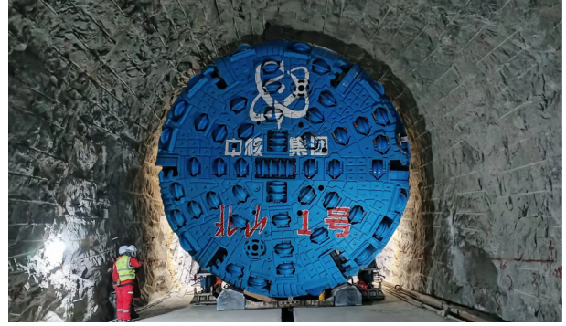
Fig. 7 The “Beishan No. 1” TBM stepping into the ramp (sourced from Wang et al. (2023)).
