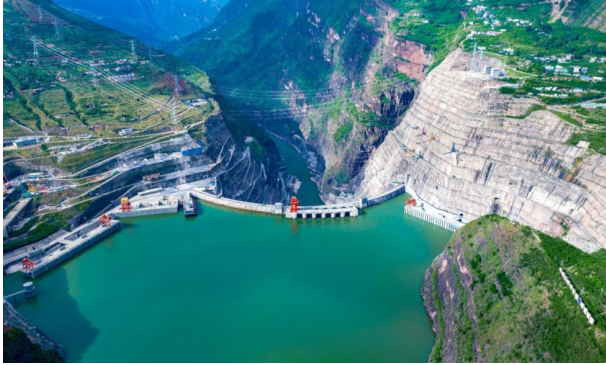
Fig. 1 Panorama of Baihetan Hydropower Station.
