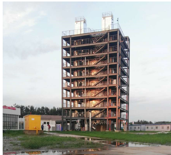
Fig. 3 Comprehensive test device of HPR1000 containment.
