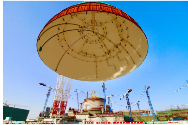
Fig. 5 Containment dome lifting of HPR1000 25 days ahead of schedule.
