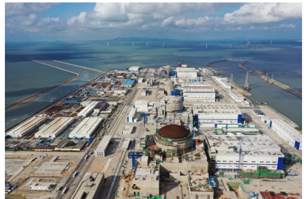
Fig. 1 Panorama of the FOAK demonstration project — HPR1000.
