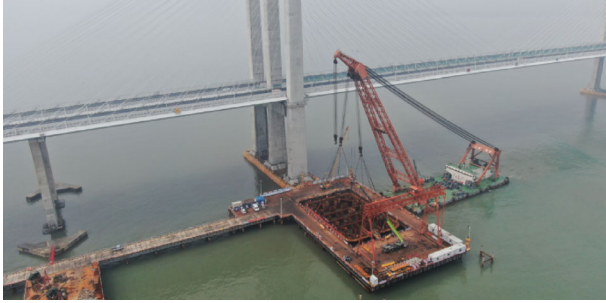
Fig. 3 Lowering of the steel suspension box of main pier.
