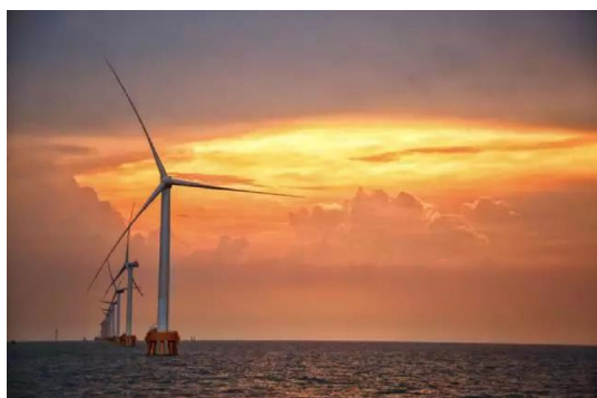
Fig. 9 Huaneng Rudong Baxianjiao Offshore Wind Farm.
