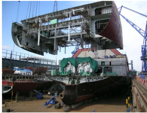
(b) Lifting of the engine room block
