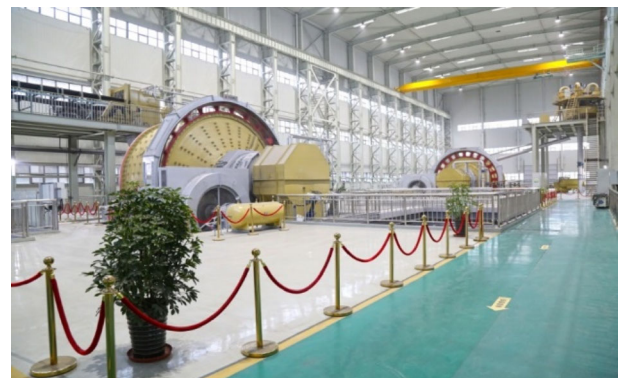
Fig. 2 Grinding Workshop of Guojiaogou Lead-Zinc Mine of Jinhui Mining Industry in Gansu Province.
