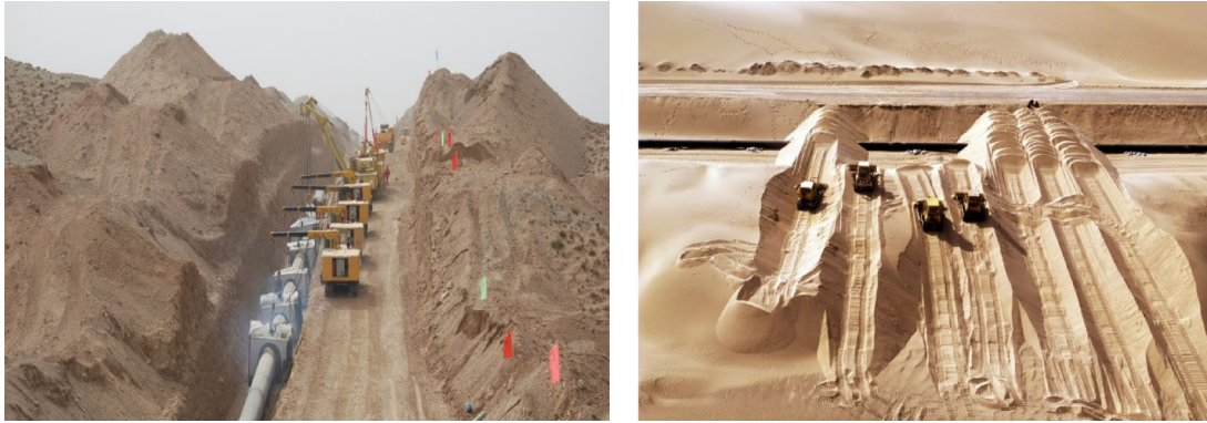
Fig. 2 Pipeline mechanized construction.
