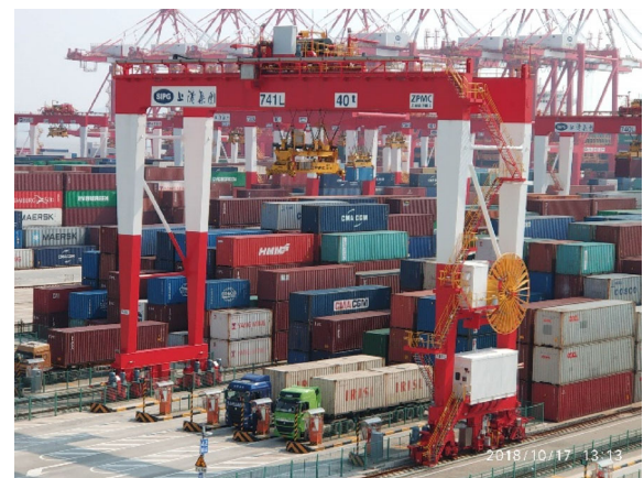
Fig. 5 Automated rail-mounted gantries (ARMGs) in Yangshan phase IV.
