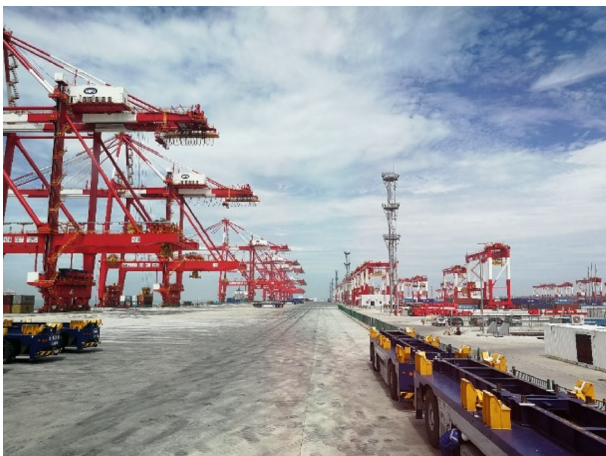
Fig. 2 The quay apron of Yangshan phase IV.
