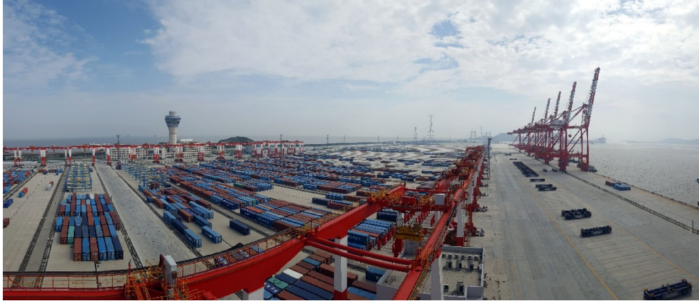
Fig. 3 A panorama of Yangshan phase IV project in equipment commissioning.
