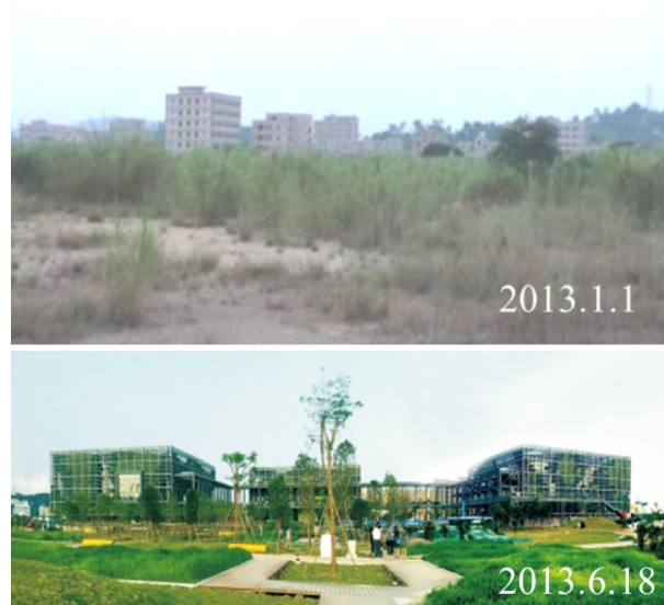
Fig. 2 Quick-start construction process of Green Workshop Reprinted from Shenzhen Institute of Building Research Co., Ltd. with permission
