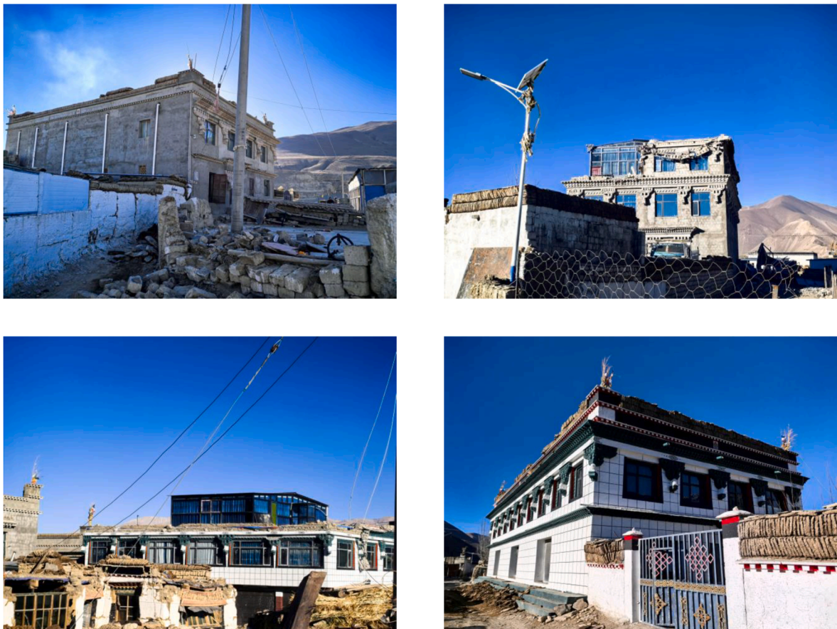
Fig. 4. Seismic damage of masonry structures with efficient seismic resistant measures.
