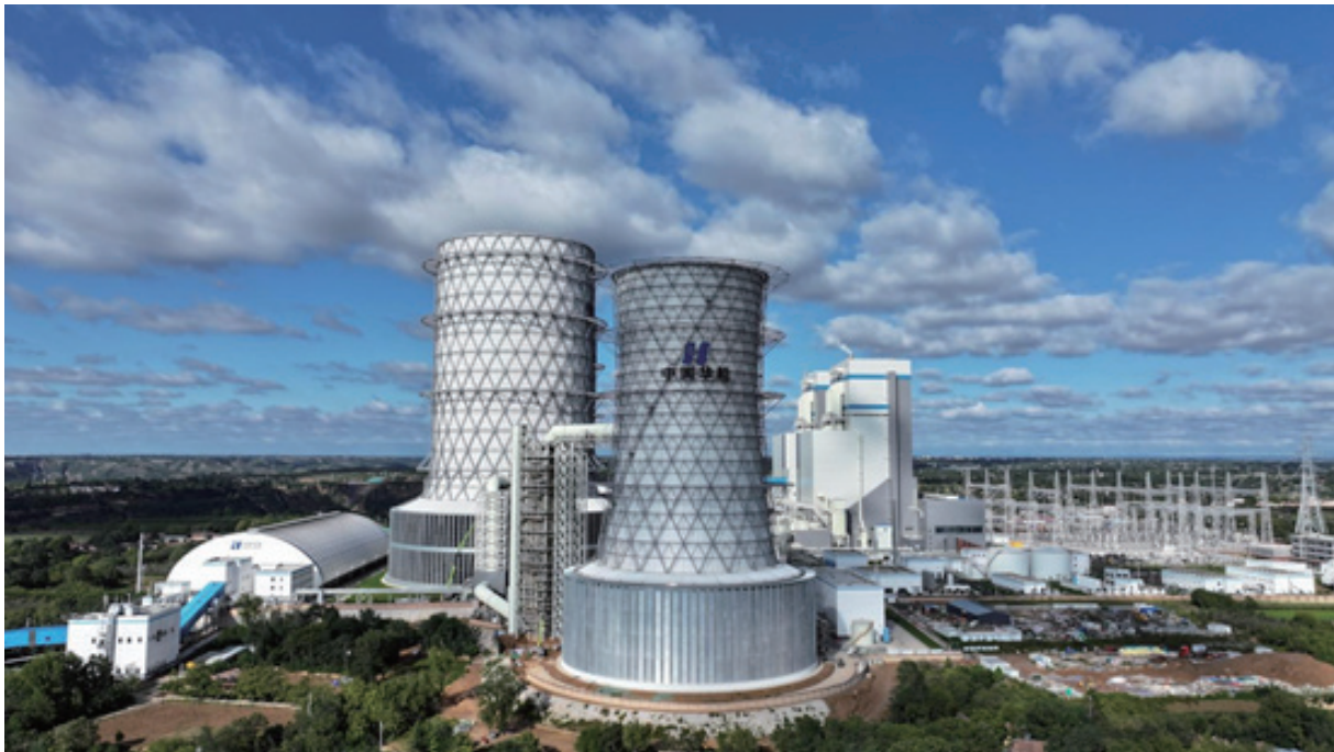
Fig. 1. Huaneng Gansu Zhengning Power Plant in Gansu Province.
