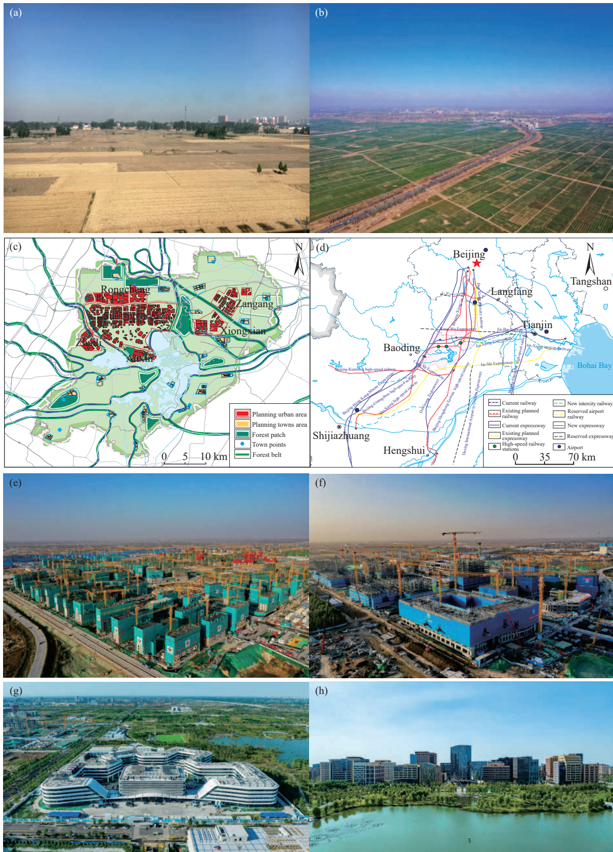
Fig. 5. Xiong'an New Area under construction. a, b—Xiong'an New Area before construction; c—map of the planning of the urban and rural spatial layout in Xiong'an New Area; d—map of the planning of regional rail transit and highways in Xiong'an New Area; e, f—Xiong'an New Area under construction (taken by Mou Yu, https://www.sohu.com/na/430127018_267106 ); g, h—city scale of Xiong'an New Area appearing.
