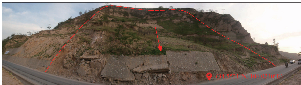
Fig. 3. Field photograph of Huanancun landslide in Tianshui City.
