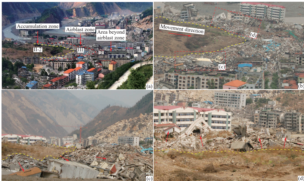
Fig. 4. Photos show the display of buildings around the Wangjiayan landslide (a) with enlarged views to show the deposited features of the collapsed buildings in the airblast zone (b–d).
