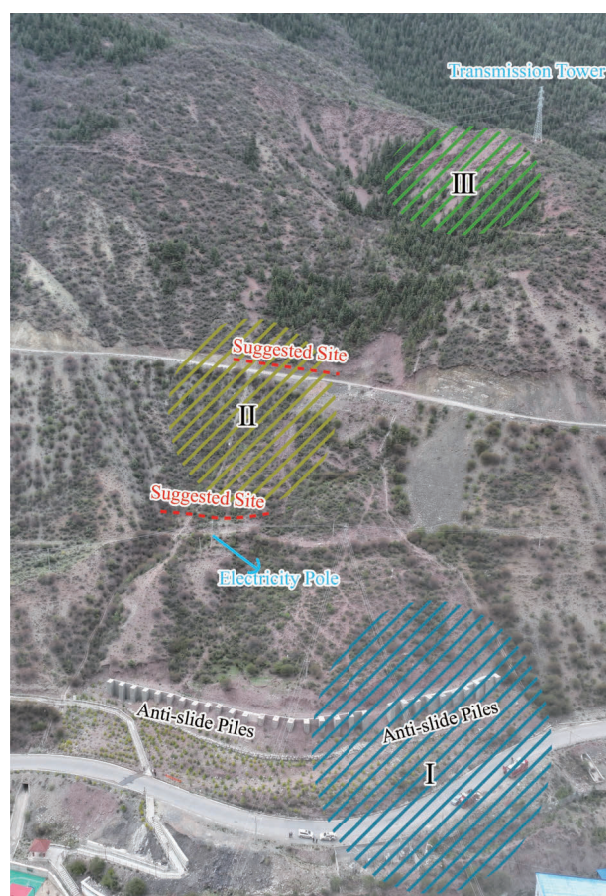
Fig. 16. Suggestion sites for anti-slide piles installation. I, II, and III correspond to area I, area II, and area III in the thickness prediction result (see Fig. 10).
