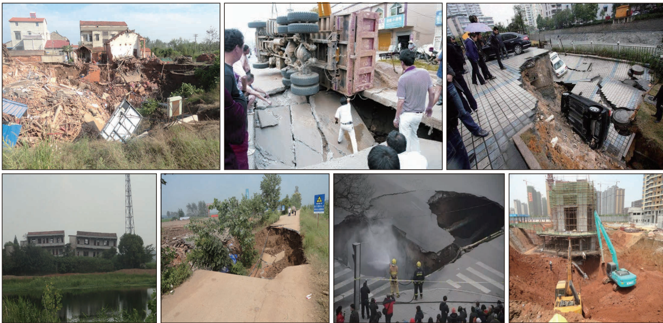
Fig. 1. Some photos of karst collapse in Wuhan City.
