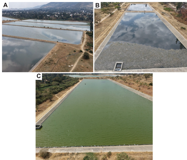
Figure 2. Kalobe waste stabilization ponds. (A) Anaerobic ponds; (B) Facultative ponds; (c) Maturation pond.
