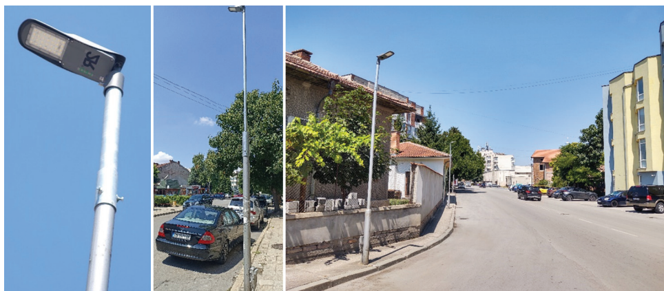
Figure 11. Photographs illustrating the technical solution involving the extension of existing park poles and the installation of street-type light-emitting diode luminaires
