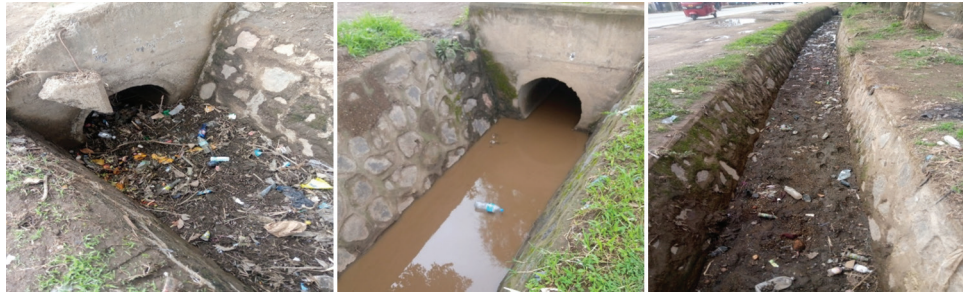
Figure 3. Photographs of the trapezoidal side drain showing (from left to right) the upstream inlet, downstream outlet, and channel approach section
