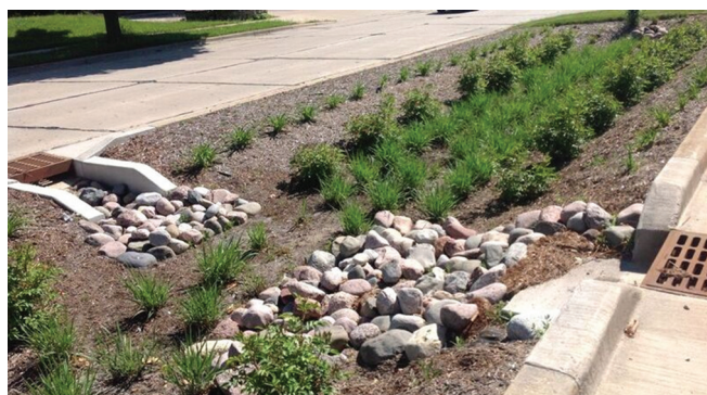
Figure 1. Filter trench in the zone of interception of polluted surface runoff
