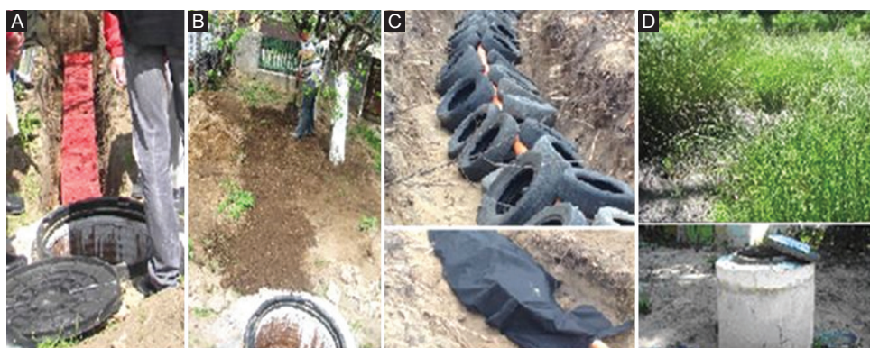
Figure 2. Sewage treatment plants for individual houses using non-traditional materials operating in Ukraine (Tatarbunary Town Museum). (A-D) Stages of filter trench construction: (A) Arrangement of a septic tank; (B) Construction of a filter trench using available space; (C) Laying waste tires and geotextiles to prevent clogging; (D) Development of a recreational area on top of the filter trench.
