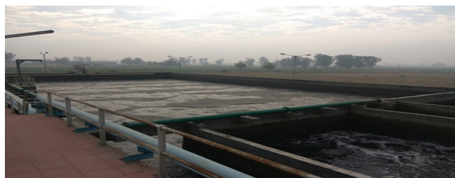
Figure 3. Sequencing batch reactor basin of the 10 mL/day sewage treatment plant at Bambianwali, Jalandhar, during the aeration and filling phase
